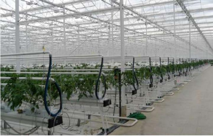
Hot water or steam leaves the boiler and is pumped into the greenhouse via a pipe network or unit heaters, or both. The pipes are typically located overhead and above the crop, or alternatively may be located beneath the benches and on the perimeter walls, or in a combination of each. Floor heating is another method to heat the greenhouse with hot water. Hot water unit heaters are another option for delivering heat into the greenhouse.
